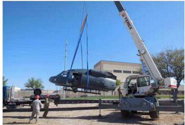
Members of the New Mexico Air National Guard 210 th RED HORSE Squadron use a crane and flatbed trailer in April to relocate a modified HH-60 helicopter airframe and training aid from the 58 th Training Squadron's aircraft yard to the DNWS training site on Kirtland AFB. The HH-60 airframe move is one of many projects that the RED HORSE Airmen are performing for DNWS, most of which are done in between other missions. (Photo by Matt Thompson, DNWS)
