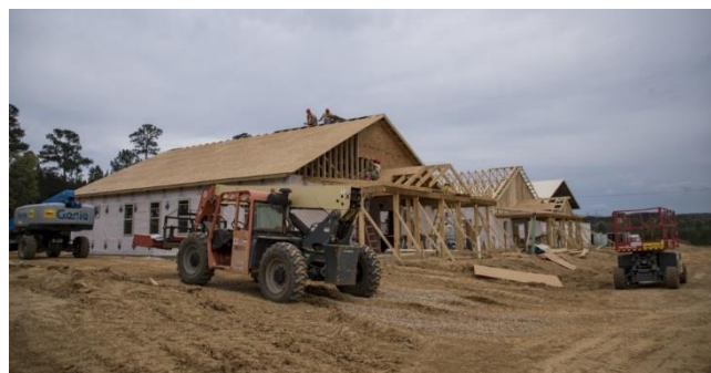
Camp Cabins being built at Camp Kamassa.
