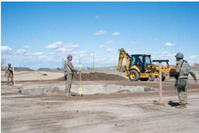
The crater profile was measured by looking between two triangles to check whether the crater is level. They filled the crater as part of the scenario.
