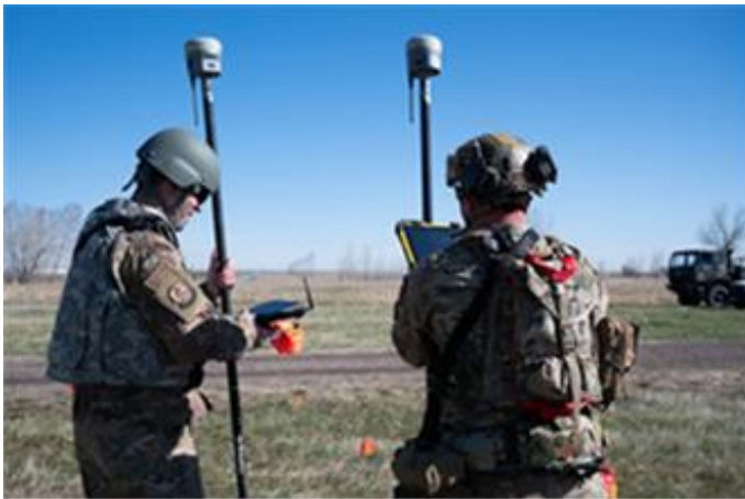
Staff Sgt. Christopher D'Amata, left, and Tech. Sgt. Benjamin Hammond, 819th RHS engineering technicians, use a survey-grade global positioning satellite device to plot the locations where structures will be built. During the exercise, squadron members built sleeping tents, shower facilities and other structures that would be necessary for a bare base in a remote location.
