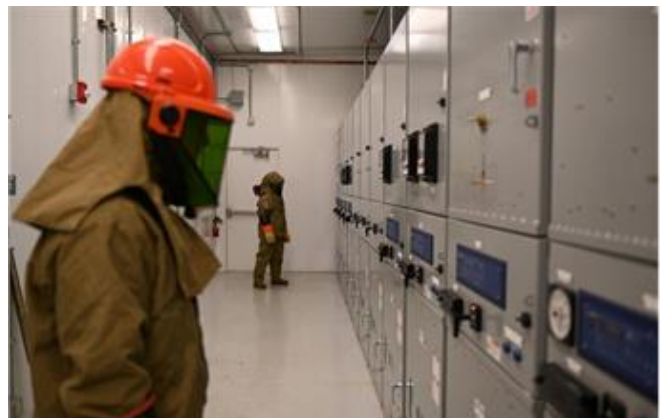
Senior Airman Tritten and Airman 1st Class Eva Enevidas, 87th CES electrical systems apprentice, prepare to shut down electrical power on Joint Base McGuire-Dix-Lakehurst as part of the ERRE training exercise.
