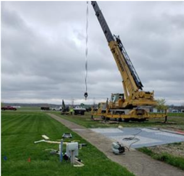
Truck arrival, preparation for offloading.
