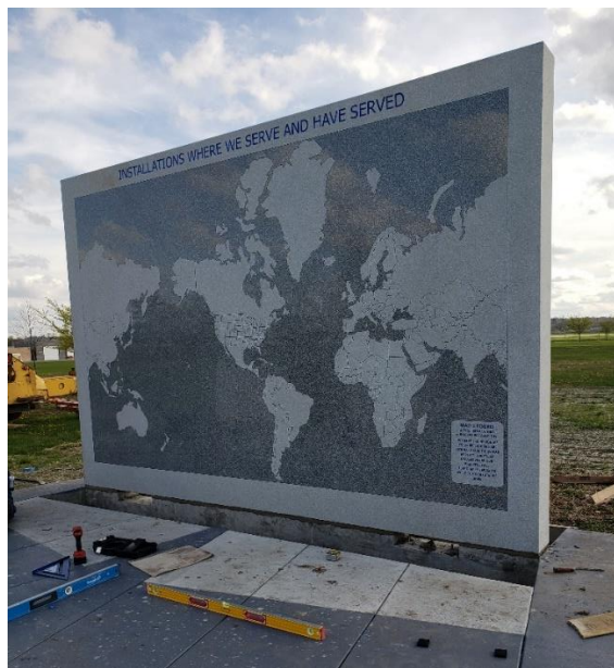
Granite slab is upright!
