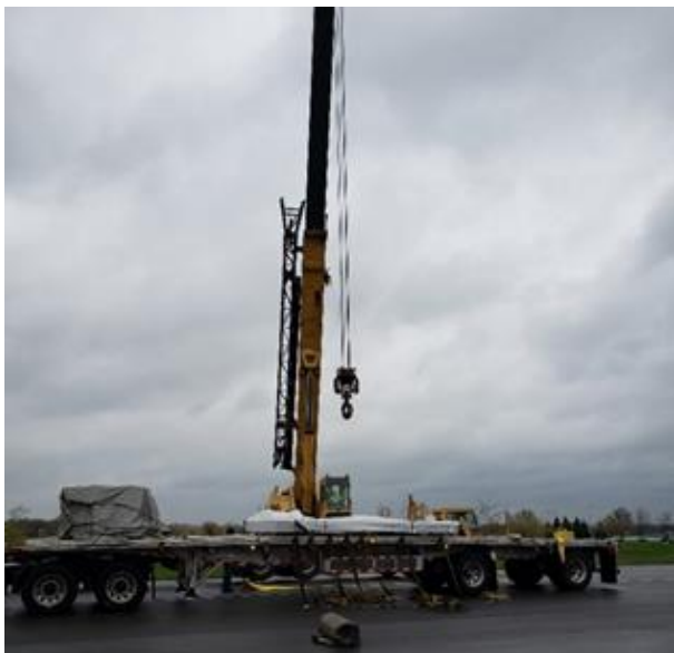
Offloading granite slab from truck bed begins.
