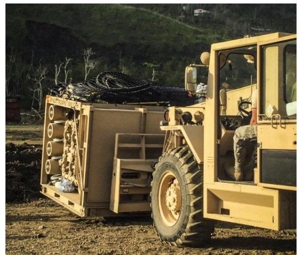
A ROWPU is being set in place to provide potable water to the local area and surrounding cities which have not had running water or electricity since Hurricane Maria made landfall.
