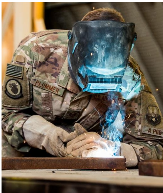
Tech. Sgt. Joshua Plummer, a water and fuels system maintenance craftsman for the 1st Civil Engineer Group's 577th Expeditionary Prime Base Engineer Emergency Force
