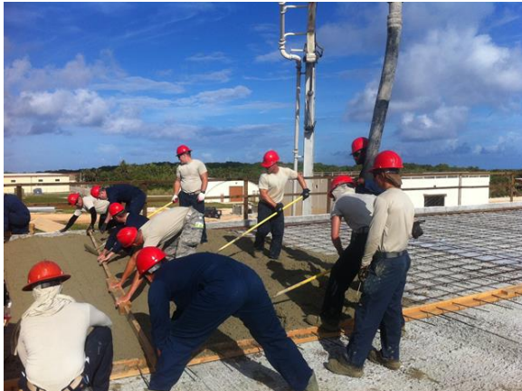
554 RHS Airmen placing 3 inch concrete topping on a Double Tee roof.
