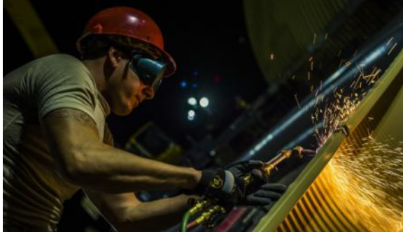
Staff Sgt. Jesse Mitchell, 557th Expeditionary RED HORSE Squadron pavement and equipment operator, cuts a metal structure with a blow torch Aug. 3, 2014, at an undisclosed location in Southwest Asia. Airmen from the 557th ERHS came from Al Udeid to build two K-Span buildings to establish more permanent structures than the current tents used as passenger terminals. The unit is comprised of all Air National Guard members deployed from PA. in support of Operation Enduring Freedom.
