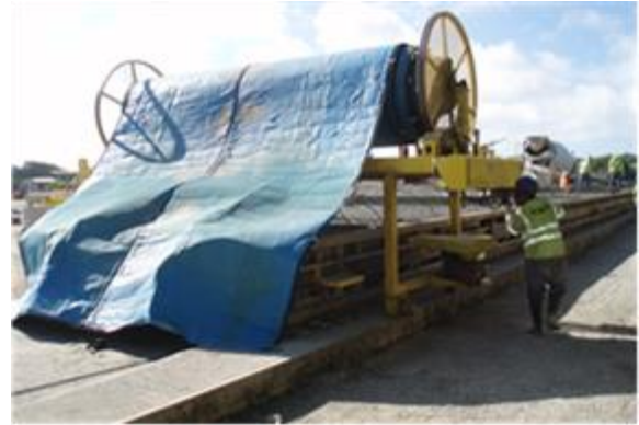
Curing blanket to create a controlled curing environment.
