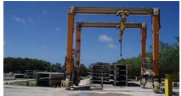
An overhead crane lifting the cured double tee beam.
