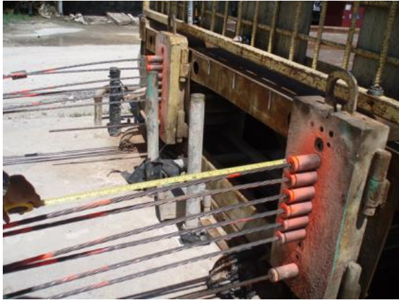
Forms for double tees are prepared with reinforcing steel.
