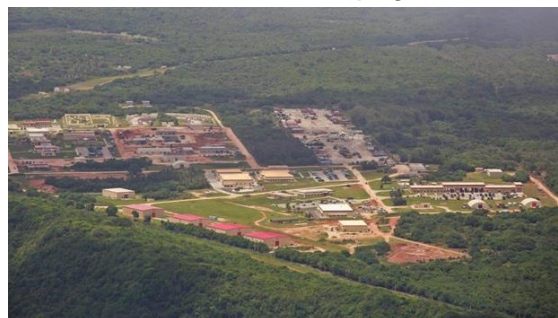
The Construction of the PACAF Regional Training Center by RED HORSE Airmen in June 2014.
