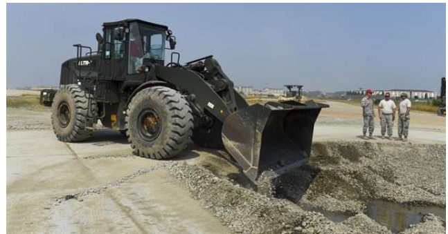
U.S. Air Force Senior Airman Robert McIntosh, 8th Civil Engineering Squadron pavement and construction journeyman, pushes gravel into a crater using a loader at Kunsan Air Base, Republic of Korea, June 23, 2017. The 8th Civil Engineering Squadron participated in airfield damage repair training as part of the final Exercise Silver Flag training held at Kunsan.
