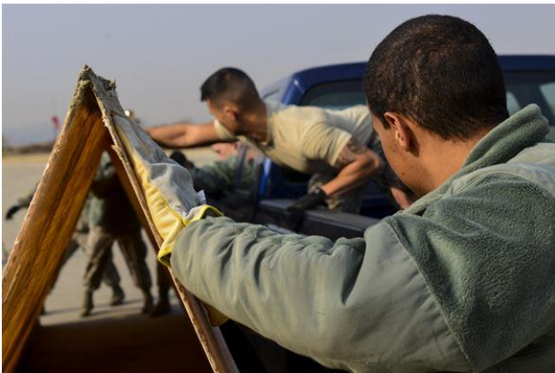
Airmen from the 51st Civil Engineer Squadron structures flight consolidate a folded fiberglass matt during Prime BEEF Day at Osan Air Base. Folded fiberglass matts are used to help reinforce damaged runways during contingency operations, with the ability to withstand the weight of a landing aircraft without fracturing.
