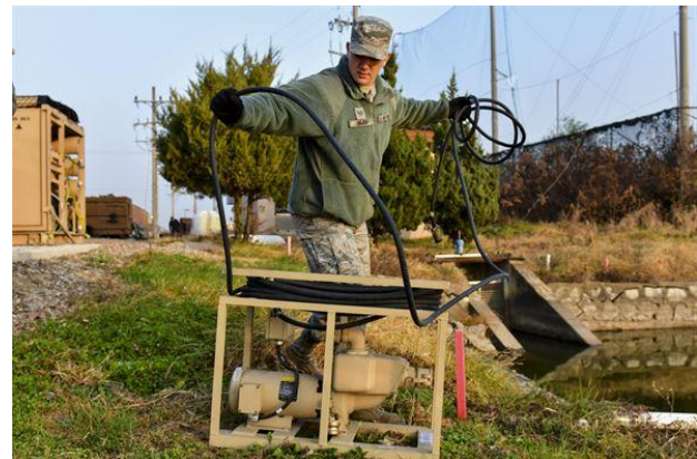
U.S. Air Force Staff Sgt. James Wajda, 51st Civil Engineer Squadron water fuels systems maintenance craftsman, sets up a raw water pump at Osan Air Base, Republic of Korea, Nov. 17, 2016. The pump is used to push water into a filtration system to generate large quantities of drinkable water for the base population.
