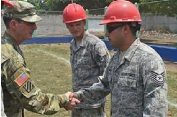
U.S. Army Lt. Gen. Joseph DiSalvo, left, U.S. Southern Command military deputy commander, shakes hands with Pennsylvania Air National Guard Tech. Sgt. Joseph Bonamico, 201st RED HORSE structures technician, outside the construction site of the new medical clinic.
