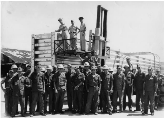
Colonel William F. Dolby, 2nd Air Division Director of Civil Engineering, tightens the last bolt to complete the steel revetments constructed by the ADC PRIME BEEF Team at Tan Son Nhut Air Base, Vietnam. Watching are Lt Col Francis E Torr, Commander of PRIME BEEF SEA and Lt Col William O. Boorman, Tan Son Nhut Base Civil Engineer. Members of ADC PRIME BEEF Team below.
