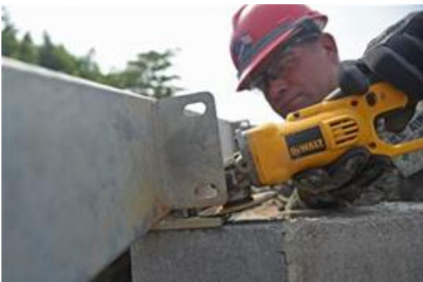
Pennsylvania Air National Guard Senior Master Sgt. Ronald Hinsey, 201st RED HORSE structures superintendent, grinds a mounting plate to size for a new medical clinic May 3, 2016 during Exercise BEYOND THE HORIZON 2016 GUATEMALA. The mounting plate is shaped to fit precisely with the truss beam and provides a flush fitting connection.
