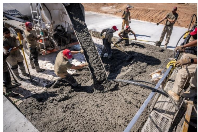
1 st ECEG Airmen pour more than 12,000 cubic meters of concrete.
