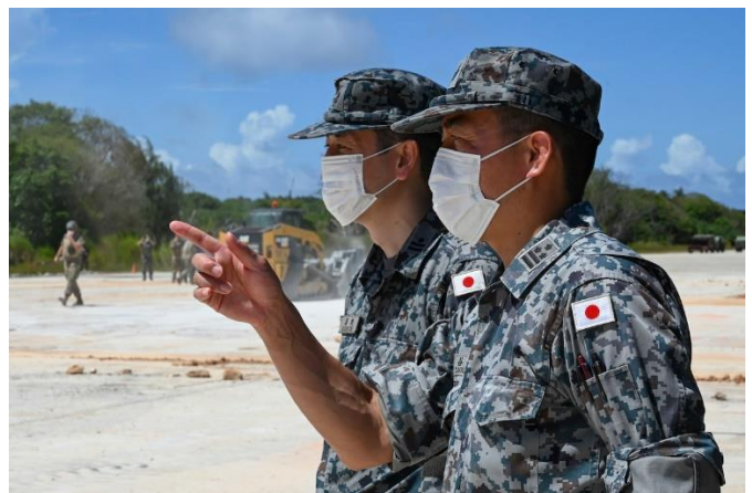
Members from the Japan Air Self-Defense Force observe the repair of an airfield runway.
