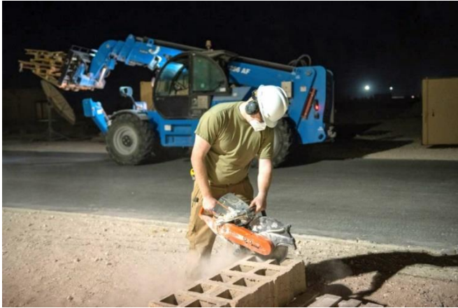
U.S. Air Force Senior Airman Alexander Mashburn, a structural journeyman with the 1 st ECEG, cuts concrete masonry units. CMUs must be cut according to very specific measurements in order to fit properly on structures being built.
