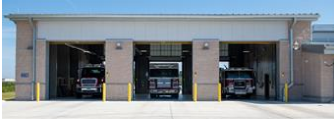
The 325th Civil Engineer Squadron's emergency response vehicles sit idle in the new Fire Station #2 at Tyndall. The station is the first building to be reconstructed after devastating damage from Hurricane Michael in 2018.
