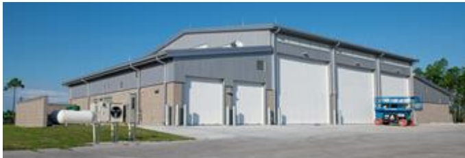
The fire contingency training facility nears completion at Tyndall. The facility will house the 801st RED HORSE Training Squadron and their emergency response vehicles, used to train members across the Department of Defense.
