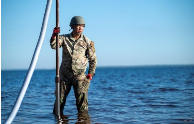
U.S. Air Force Tech. Sgt. Kevin Ilano, 45th Civil Engineering Squadron structural craftsman, anchors a pipe during a water filtration event April 23. (U.S. Space Force photo by Airman 1st Class Spencer Contreras).
