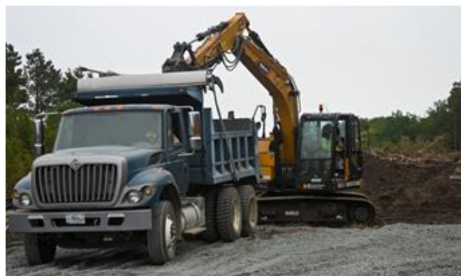
Pennsylvania Air National Guardsman, Senior Airman John Trimbath, assigned to the 171st CES, loads debris into a dump truck while operating an excavator during the deployment.
