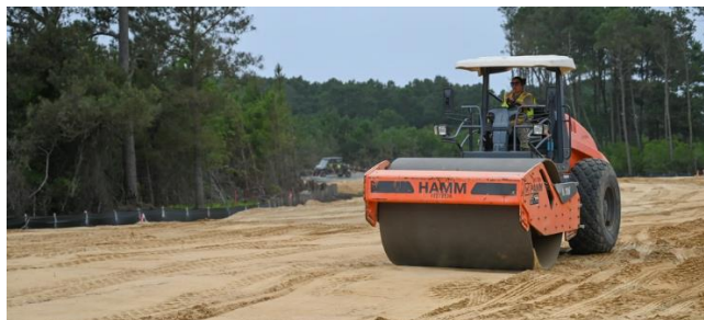
Tech. Sgt. Mary Connelly, assigned to the 171st CES, operates a road roller to create a compact driving surface for other vehicles during the deployment to Assateague Island for training.
