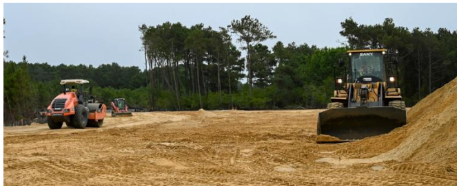
Pennsylvania Air National Guardsmen assigned to the 171st Air Refueling Wing spread and compact sand fill as a foundation for a parking lot during the deployment to Assateague Island.
