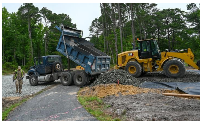
A team of 171st Civil Engineers assigned to the Pennsylvania Air National Guardsman, operate a dump truck to deliver a load of riprap while a front loader spreads it out during the deployment.
