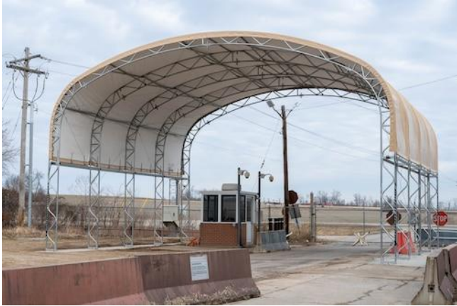
An overhang, developed by Airmen from the 375th Civil Engineer Squadron, stands over the Cardinal Creek Gate on Scott Air Force Base, Illinois, 25 February 2026. The overhang provides defenders protection from the elements, reducing weather-related gate closures and improving overall working conditions while helping sustain operations during inclement weather. (U.S. Air Force photos by Staff Sgt. Stephanie Henry)
