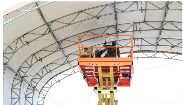
Airmen from the 375th Civil Engineer Squadron install lights on the overhang that stands over the Cardinal Creek Gate on Scott Air Force Base, Illinois, 25 February 2026. The overhang provides defenders protection from the elements, reducing weather-related gate closures and improving overall working conditions while helping sustain operations during inclement weather. (U.S. Air Force photos by Airman 1st Class Devin Morgan)
