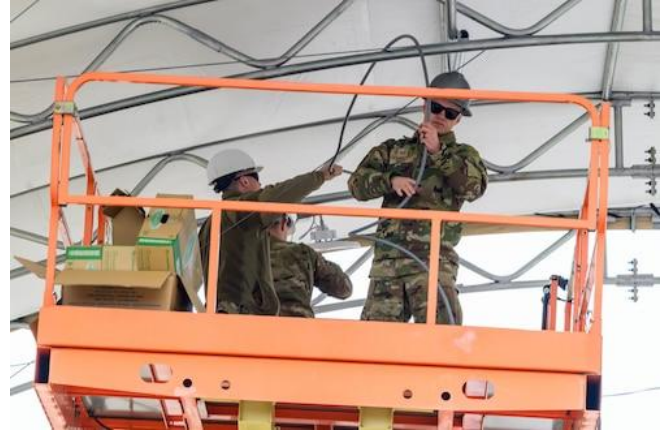
Airmen from the 375th Civil Engineer Squadron install lights on the overhang that stands over the Cardinal Creek Gate on Scott Air Force Base, Illinois, 25 February 2026. The overhang provides defenders protection from the elements, reducing weather-related gate closures and improving overall working conditions while helping sustain operations during inclement weather. (U.S. Air Force photos by Airman 1st Class Devin Morgan)
